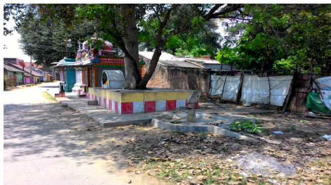
Figure 2: Location of Bore Well 6
